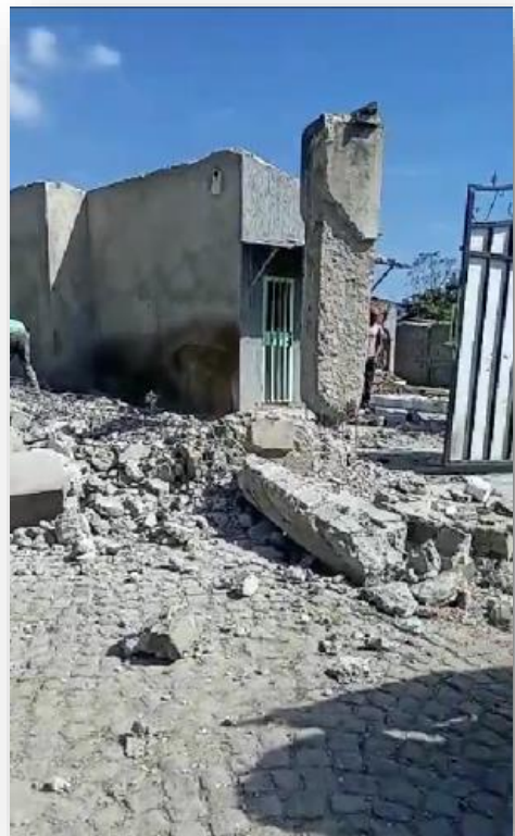
The demolition is in full
